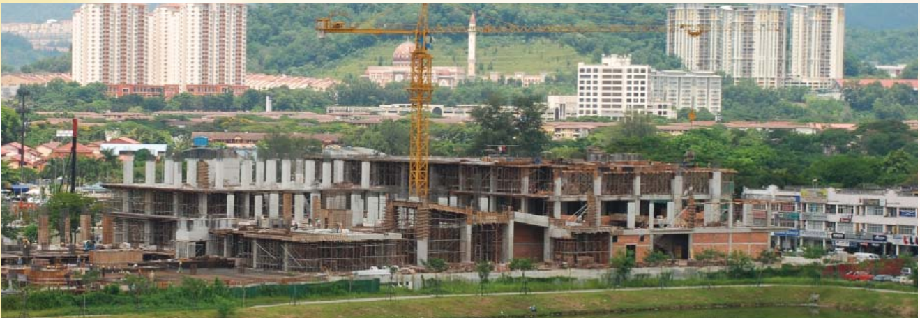
View of project job site
