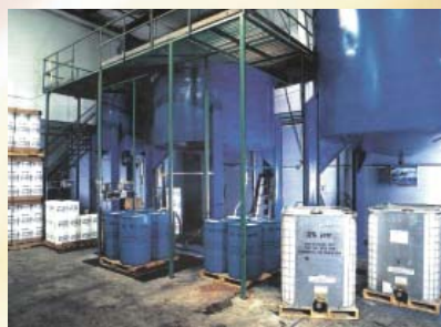
Chemguard FOAM SYSTEM - UL Approved Sole foam blending facility in South East Asia and serves as "National Disaster Response Center"
