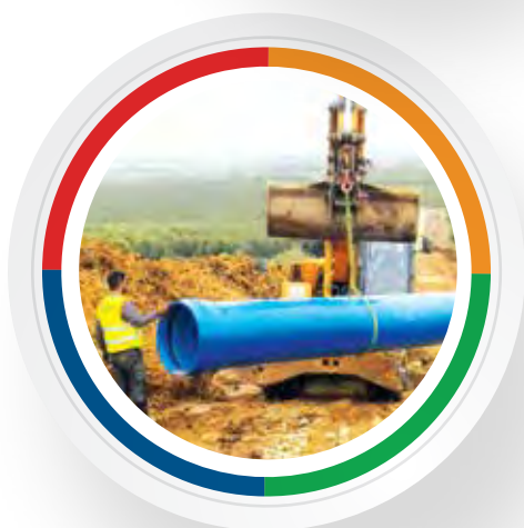
PVC-O DN800 installation (Spain)
