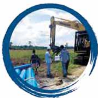
HYPRO® PVC-O for paddy granny irrigation project in Sarawak
