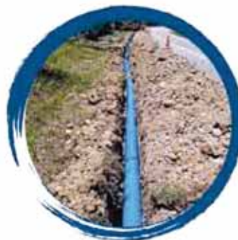
HYPRO® PVC-O for water supply project in Kelantan
