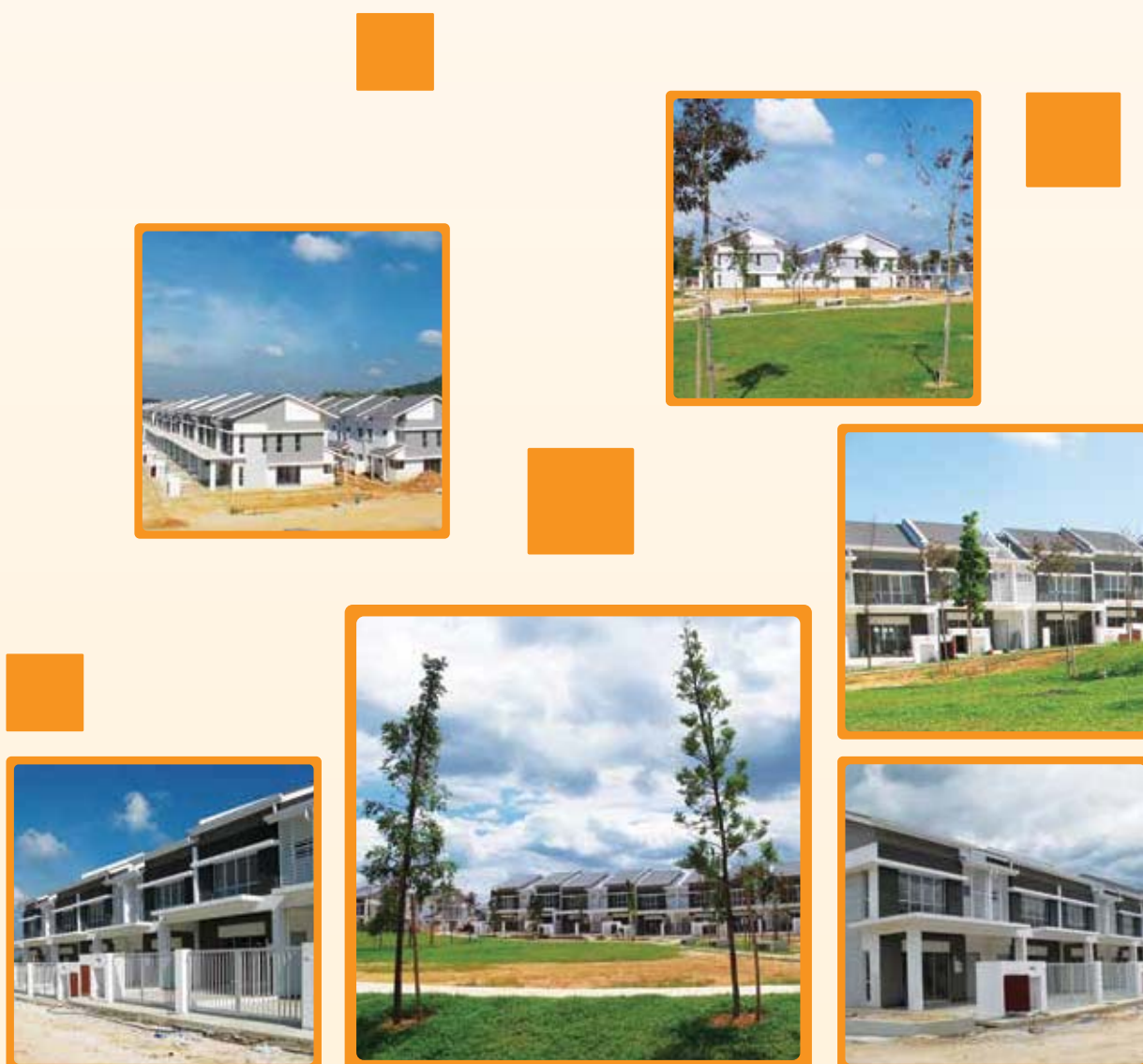
Site Construction Progress
