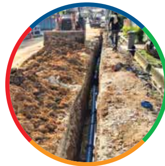
HYPRO® PVC-O for pipe replacement project in Johor
