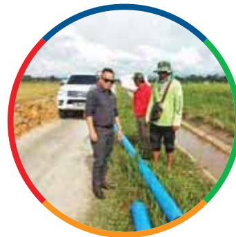
HYPRO® PVC-O for Rural Water Supply Project in Sabah
