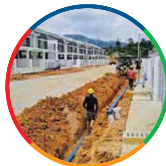
HYPRO® PVC-O pipe for water reticulation system in a private housing project in Selangor
