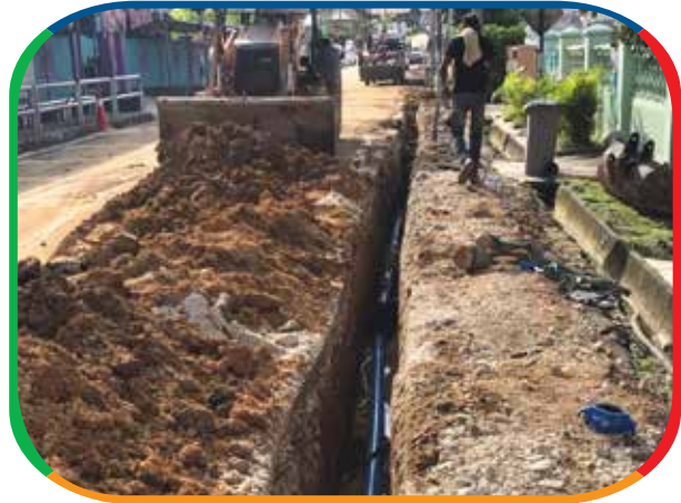
HYPRO® PVC-O for pipe replacement project in Johor
