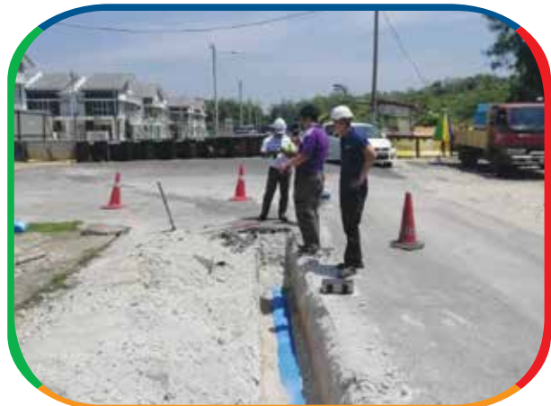
HYPRO® PVC-O pipe for water external reticulation system in a private housing project in Selangor
