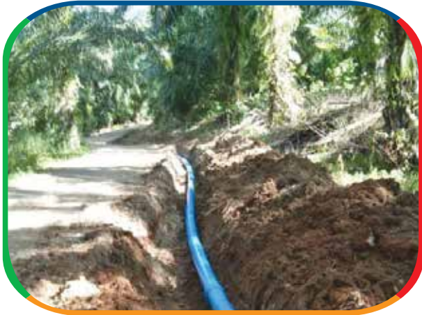
HYPRO® PVC-O for Rural Water Supply Project in Sabah
